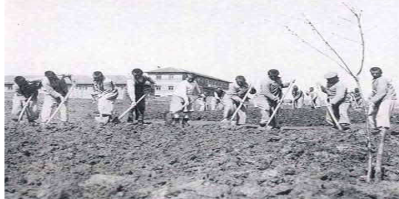
Figure 9. Students in a village institute are working in a garden
